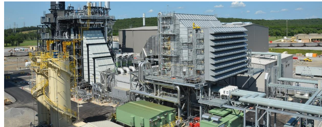
Client GRDA (Grand River Dam Authority) Plant (country) Grand River Energy Center (Americas) Generating Power 505 MW Start Up 2017
