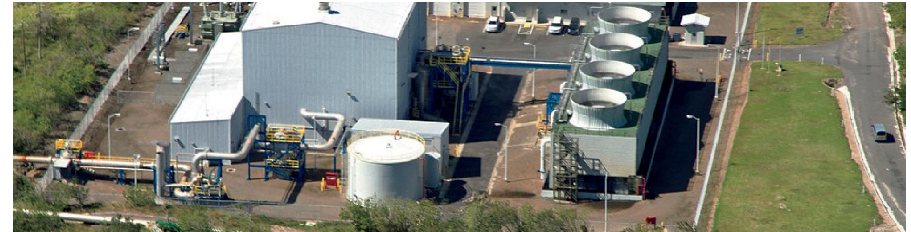
Client Instituto Costarricense de Electricidad Plant (country) Miravalles III Power Station (Costa Rica) Generating Power 27 MW Start Up 2000
