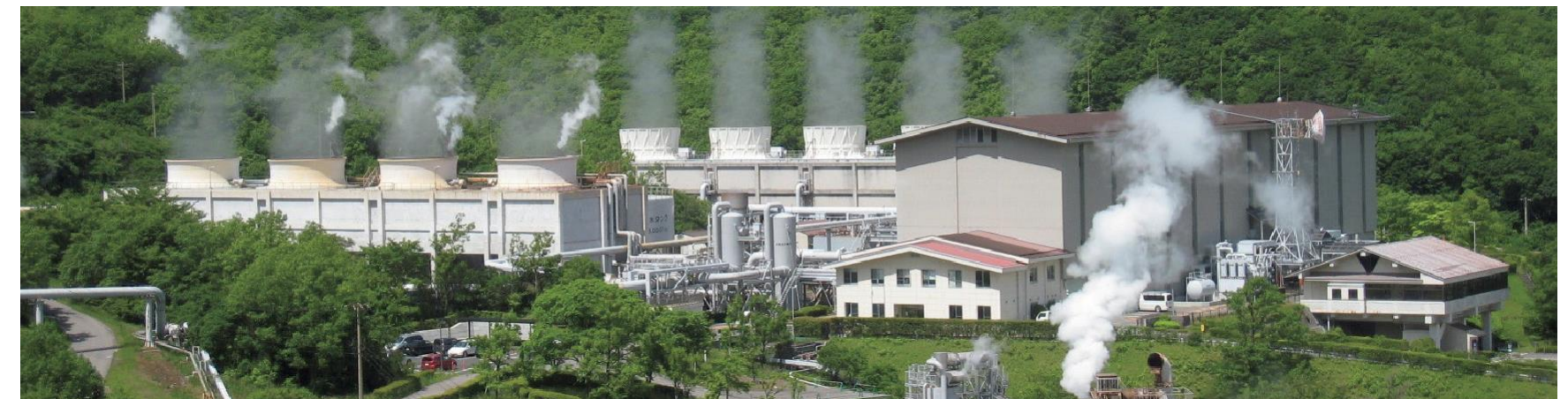
Client Kyushu Electric Power Co., Inc. Plant (country) Hatchobaru Power Plant Units 1, 2 (Japan) Generating Power 110 MW Start Up 1977 / 1990
