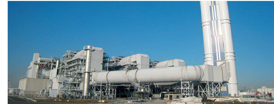
Client JERA Co., Inc. Plant (country) Kawasaki Thermal Power Station Group 1, 2 (Japan) Generating Power 3,420 MW Start Up 2009 / 2016
