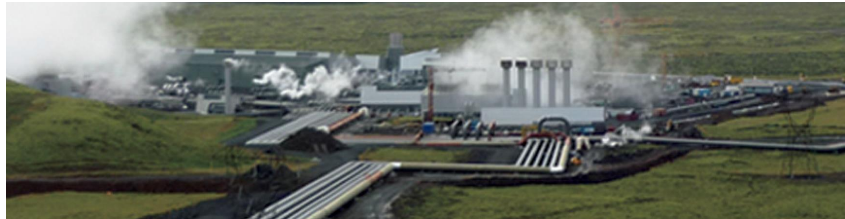
Client Reykjavik Energy Plant (country) Hellisheidi Geothermal Power Plant (Iceland) Generating Power 250 MW Start Up 2006 — 2011
