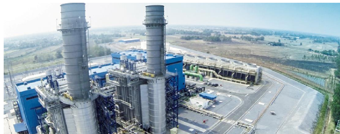
Client Gulf JP NS Company, Limited Plant (country) Nong Saeng Power Plant (Thailand) Generating Power 1,600 MW Start Up 2014
